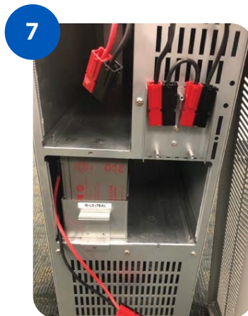
7 Install new batteries. Starting with the lowest shelf, slide in a total of 3 battery trays with battery terminals/harness facing outboard edge of the UPS.
